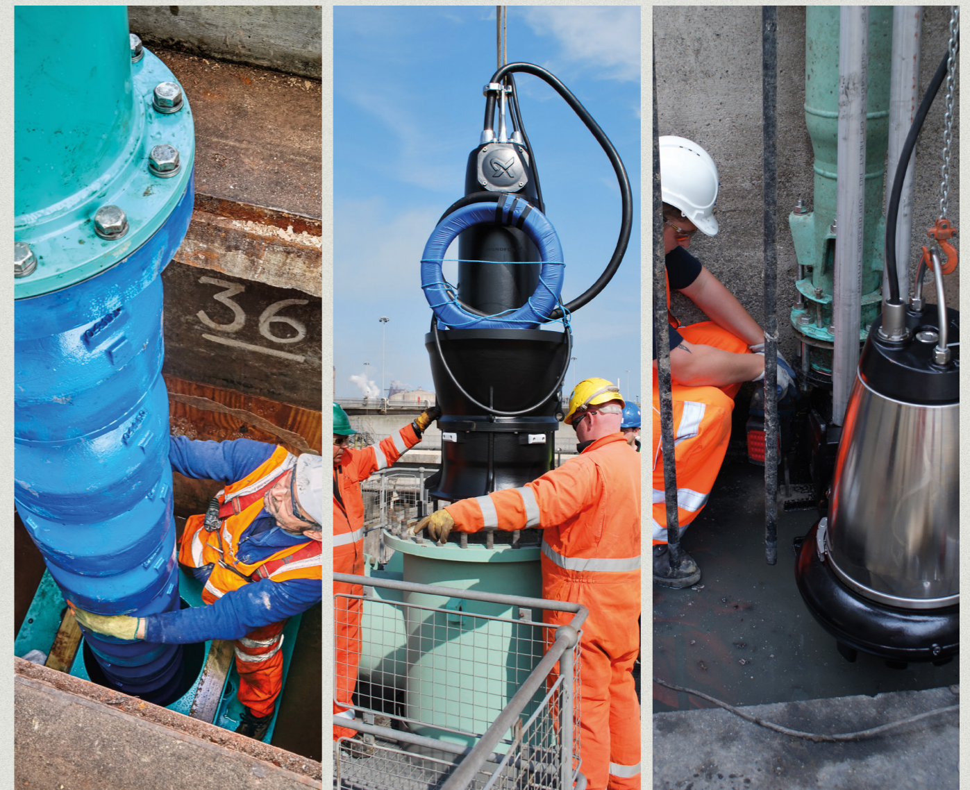
Installation of a Grundfos Peerless vertical turbine pump
