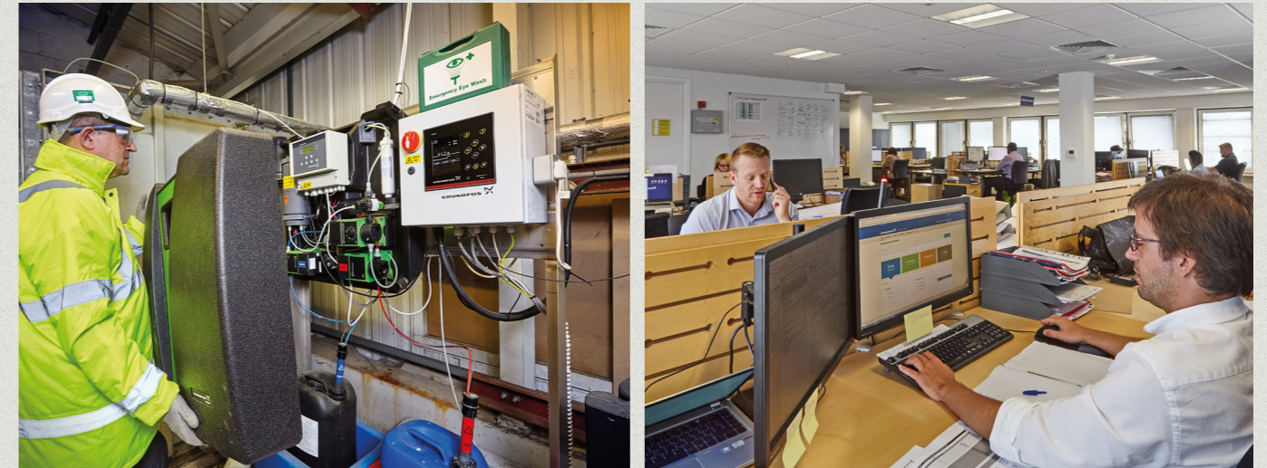
An Oxiperm disinfection unit being installed
