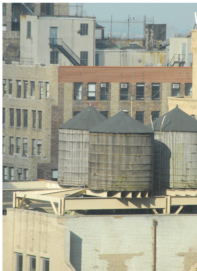
Wooden roof top tanks in New York City.
