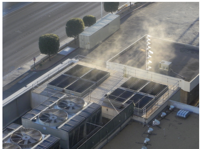
The spray from a cooling tower can easily travel 3.5 miles.
